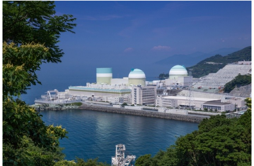
paprikaworks/iStock/Getty Images Plus Ikata nuclear power plant (Ehime Prefecture) in Japan
