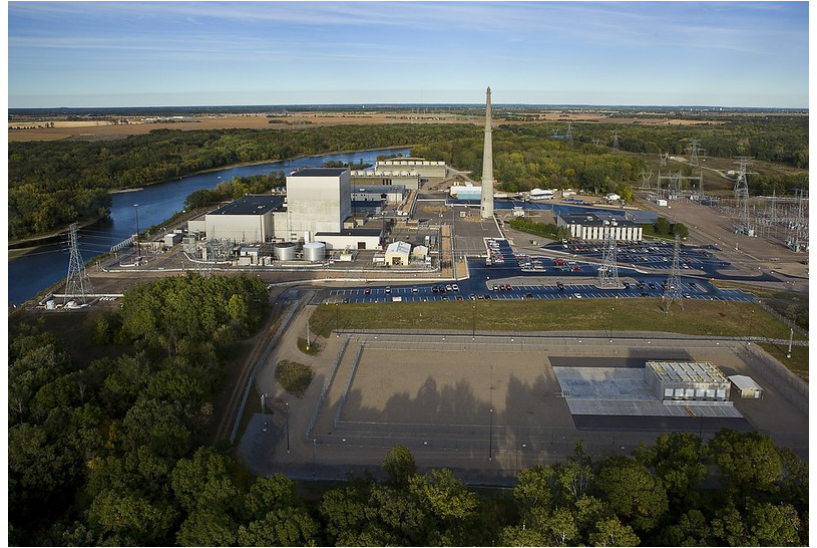
Photo courtesy of NRC Monticello nuclear plant
