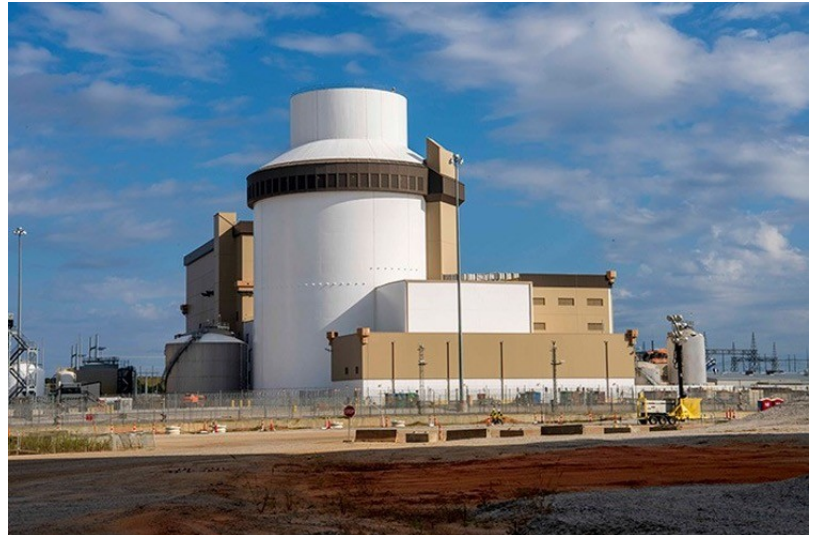
georgiapower.com Vogtle unit 3
