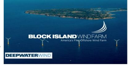
Deepwater Wind, a private energy firm, put the finishing touches on the Block Island Wind Farm in August. The five wind turbines, each 600 feet tall, were installed in the Atlantic Ocean, just off the coast of Block Island, a 10-square-mile cay situated 13 miles south of the Rhode Island mainland. The turbines are expected to begin generating electricity in November.
