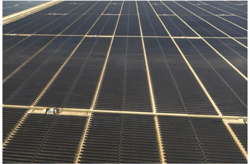
Photo of a photovoltaic solar-panel farm: kertu_ee/iStock/Getty Images Plus
