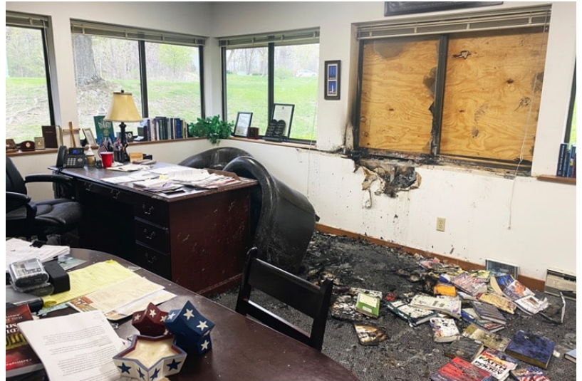
AP Images Vandalized Wisconsin Family Action office
