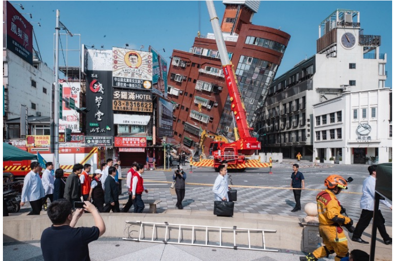
AP Images Aftermath of earthquake in Taiwan
