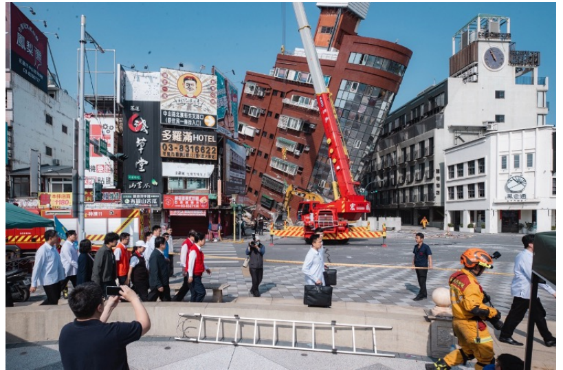
AP Images Aftermath of earthquake in Taiwan
