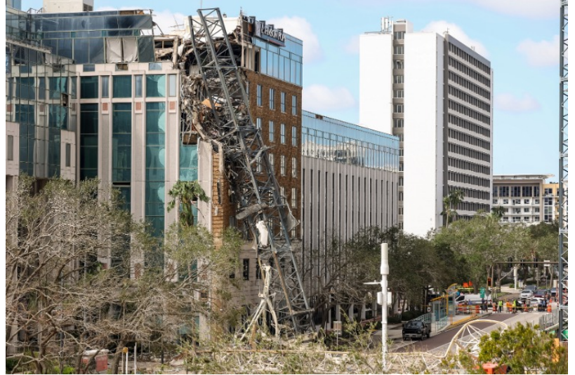
AP Images St. Petersburg after Hurricane Milton
